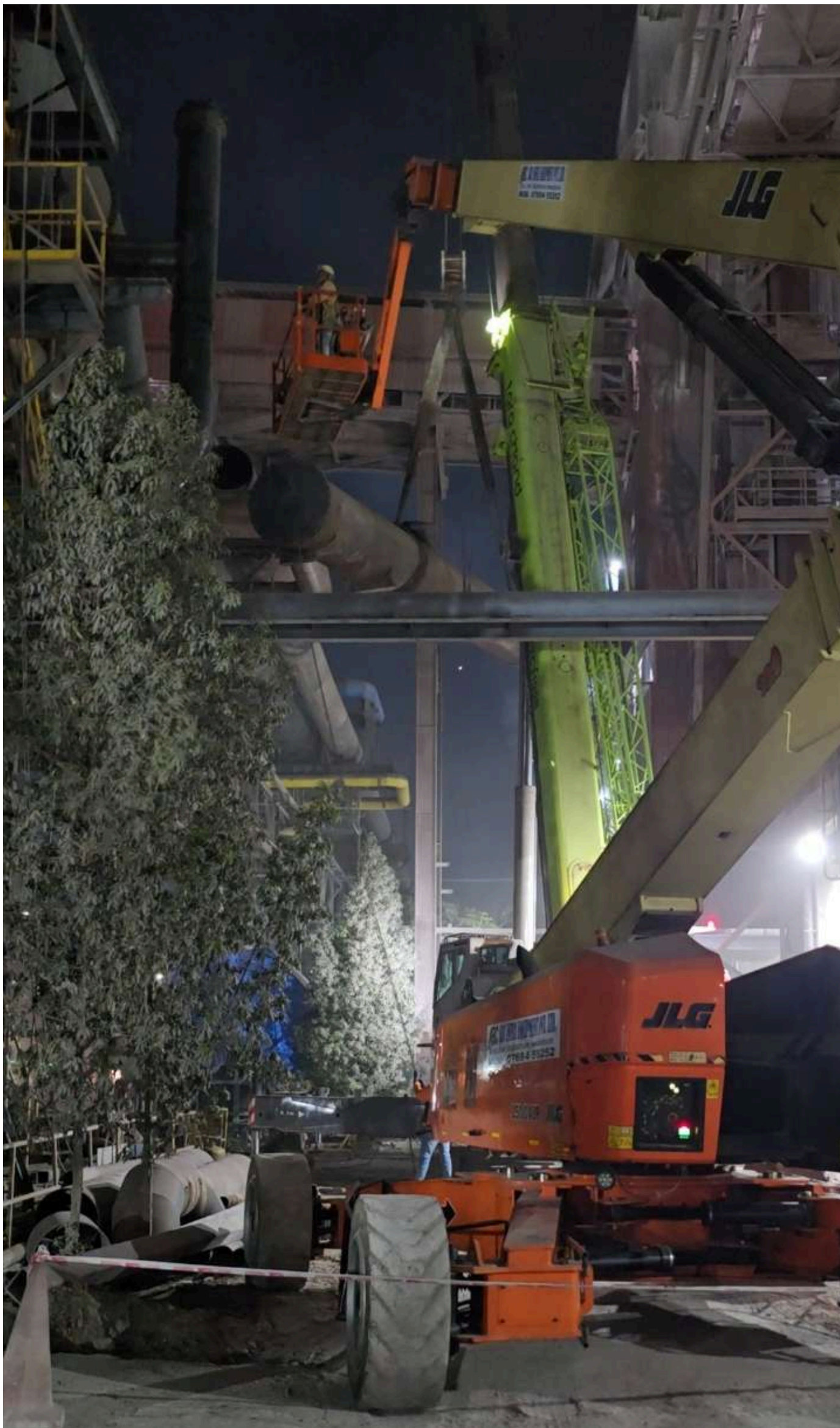
Fig.2.2: Dismantling of industrial pipe for maintenance
