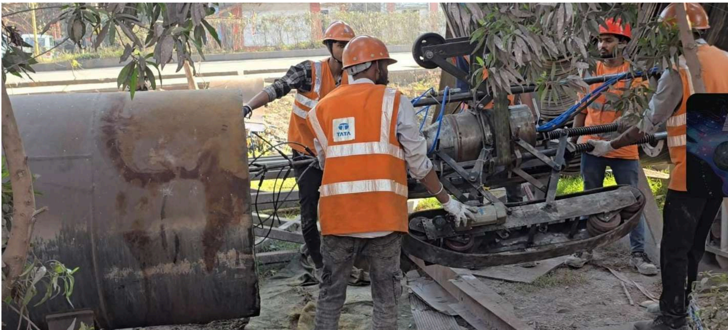
Fig. 6.4 Test run at TATA Steel Kalinganagar.
