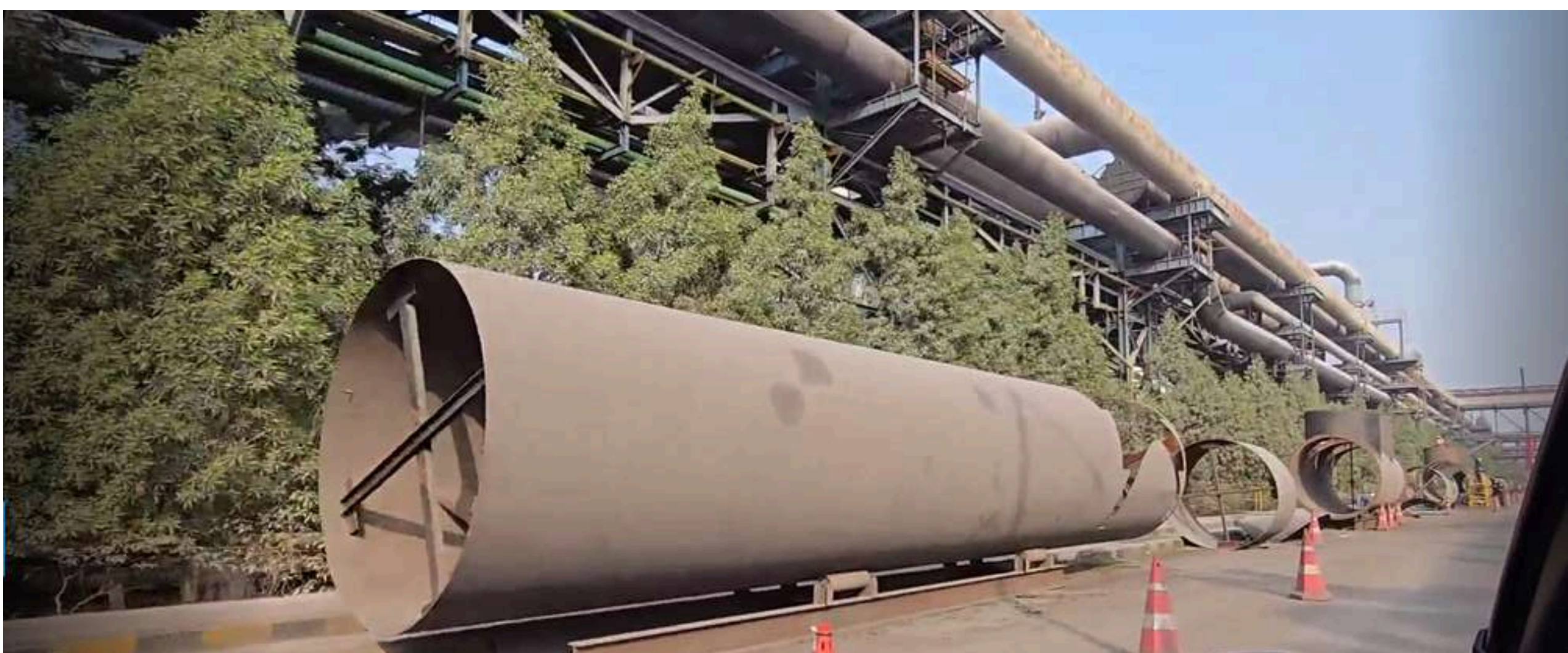
Fig.2.1: Dismantling of industrial pipe for maintenance
