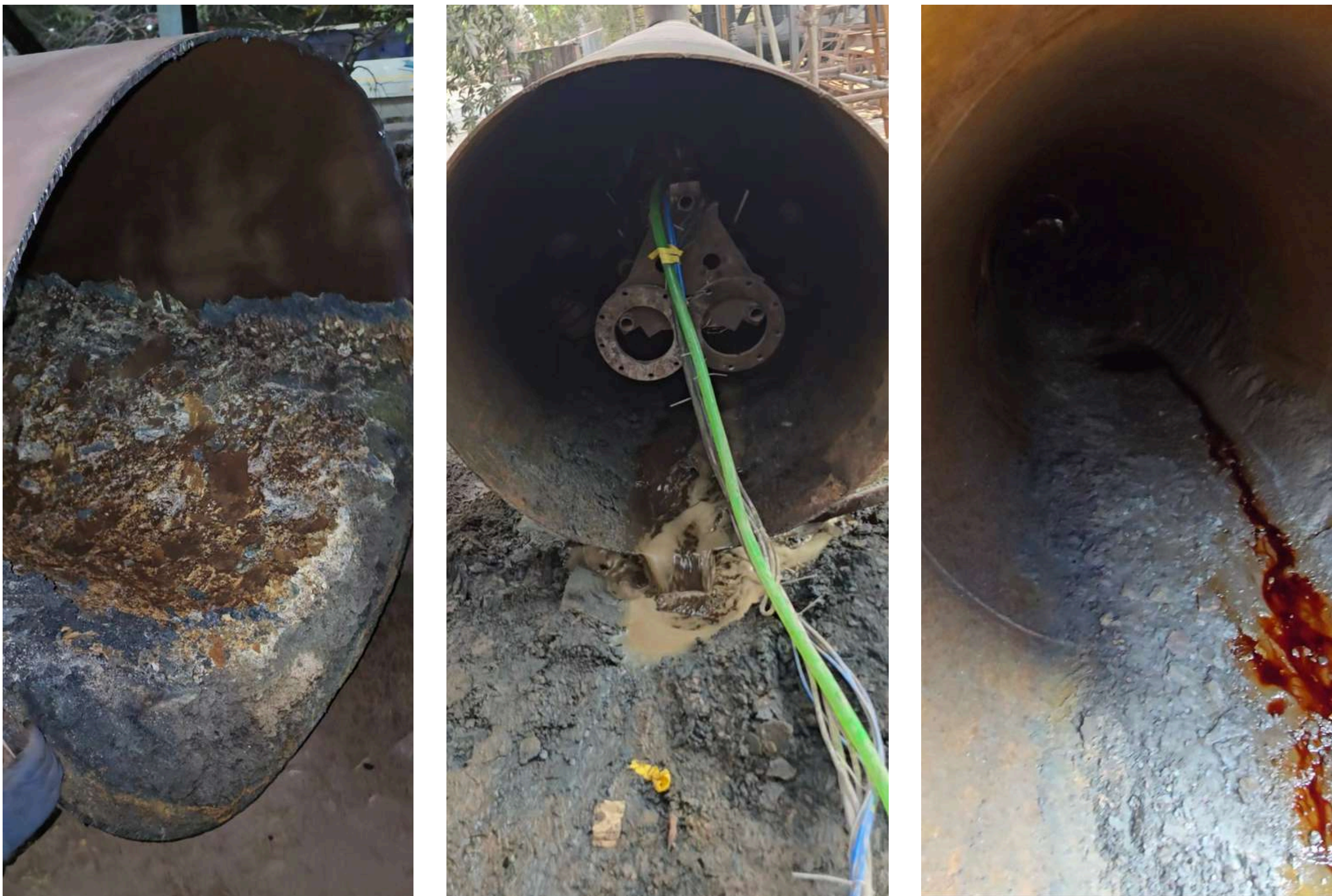
Fig.6.1,6.2 & 6.3 : Shows the before, during and after of M-TBM cleaning process at TATA Steel Kalinganagar.
