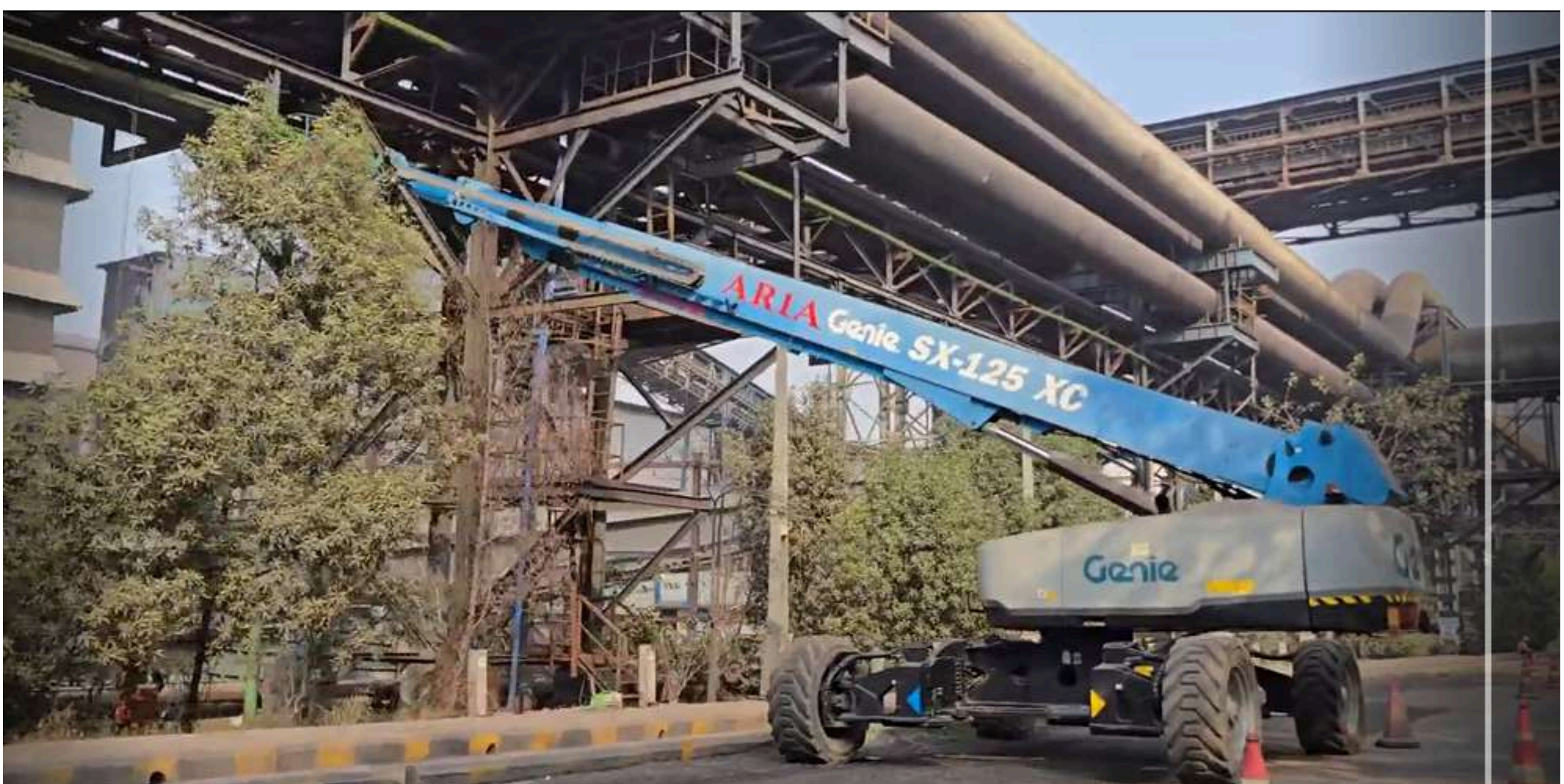
Fig.2.4: Inspection of industrial pipe for maintenance
